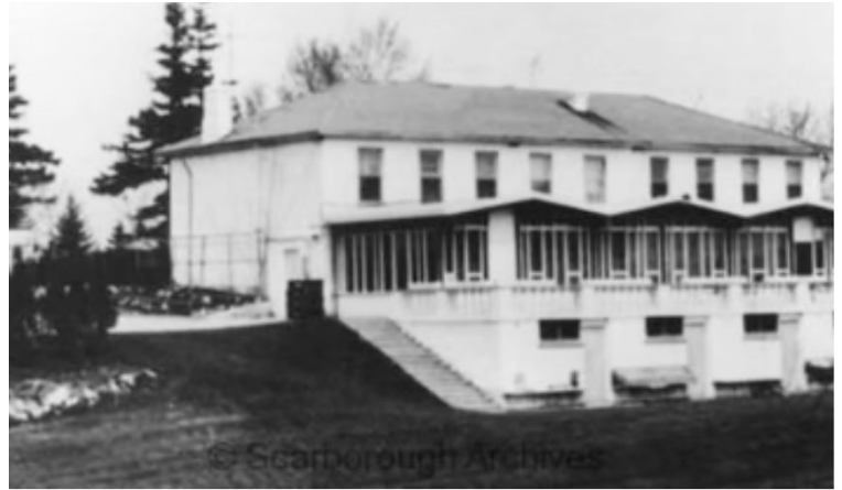
▲ Photo: Masaryktown / The Jackson farm before and after renovation & Prague Restaurant
